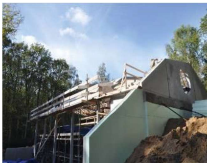
Perimeter insulation
